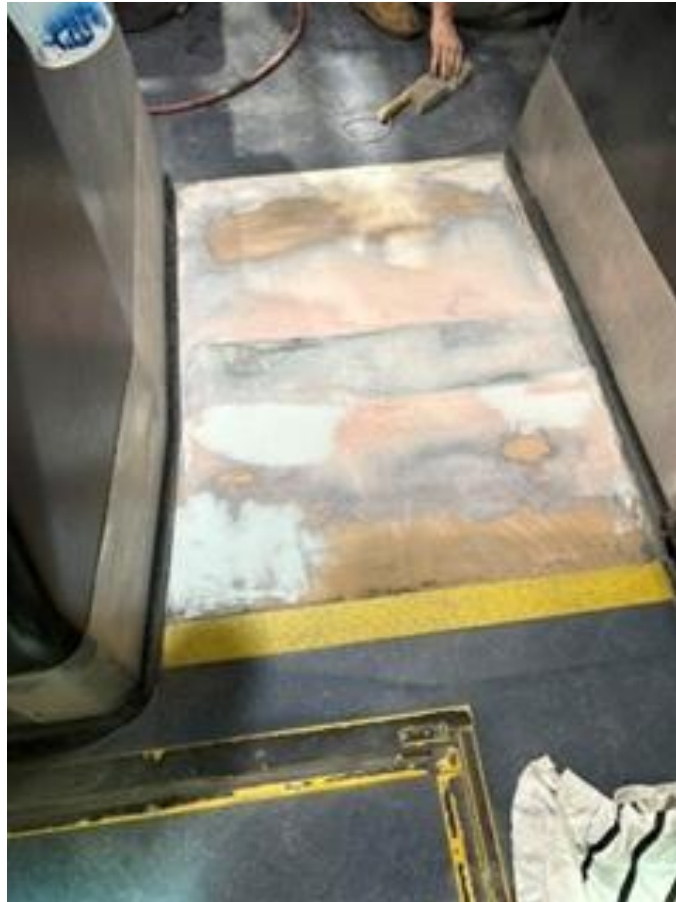
FIGURE 5 SHOWN FLOOR PREP BEFORE RE-APPLYING FLOORING
