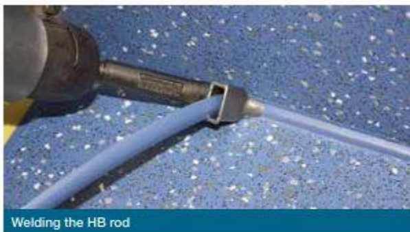
Welding the HB rod
