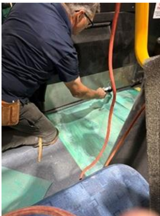
FIGURE 6: SHOWN APPLICATION OF THE 3M GLUE ON BACKSIDE OF FLOORING AND PLYWOOD SURFACE
