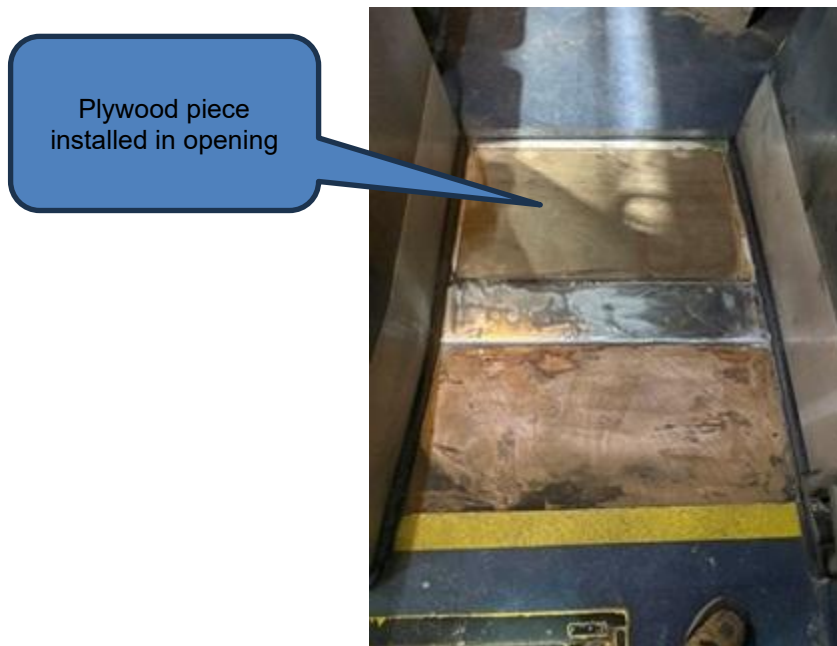
FIGURE 16: INSTALL PLYWOOD PIECE
