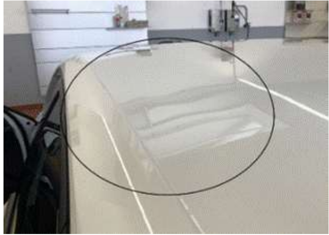
Figure 5. Surface deformations caused by large amounts of snow falling off a roof.
