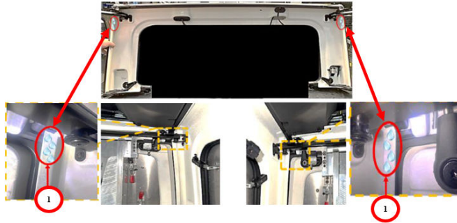
Fig. 1 Water Leak Path Indicating Weatherseal Wet-Out
