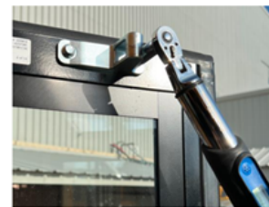
Torque to 9.7 - 10.7Nm
