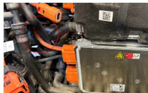
Live high-voltage line
