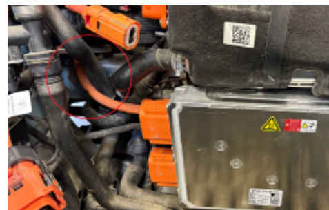
Live high-voltage line
