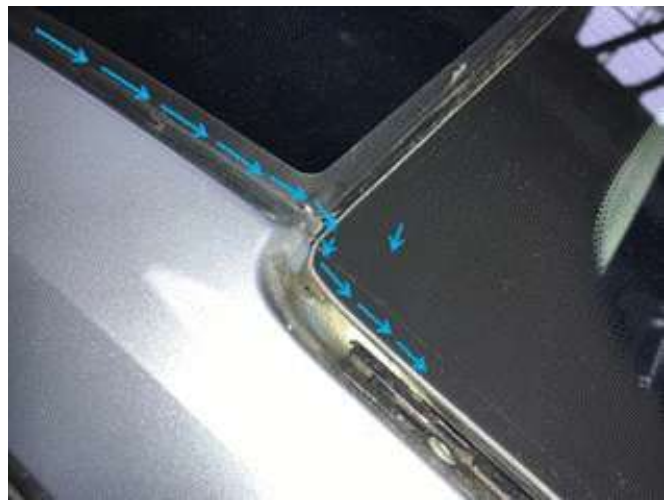
Figure 12. Drainage channels rinsed.
