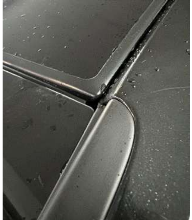
Figure 15. Water deflector reinstalled.
