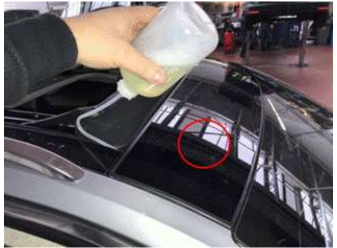
Figure 11. Rinsing the drainage channels.
