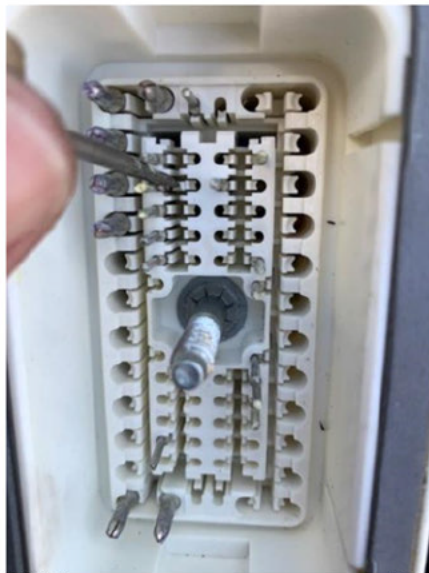
Fig. 9, Extracting the Terminal
