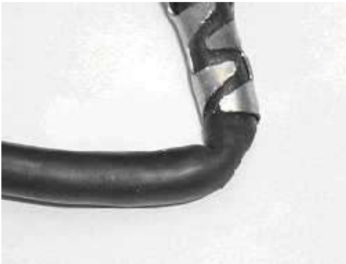
Figure 3. Copper core cracked.
