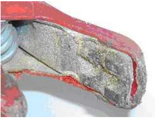
Figure 2. Oxidation on contact surface.
