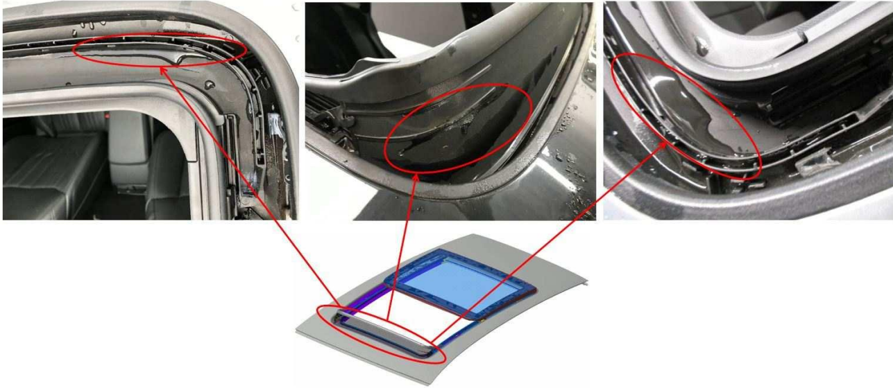
Figure 1. Examples of standing water in the wind deflector.
