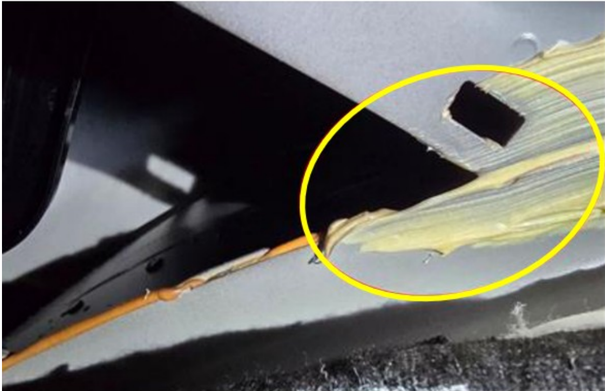
Figure 4. Excess structural adhesive
