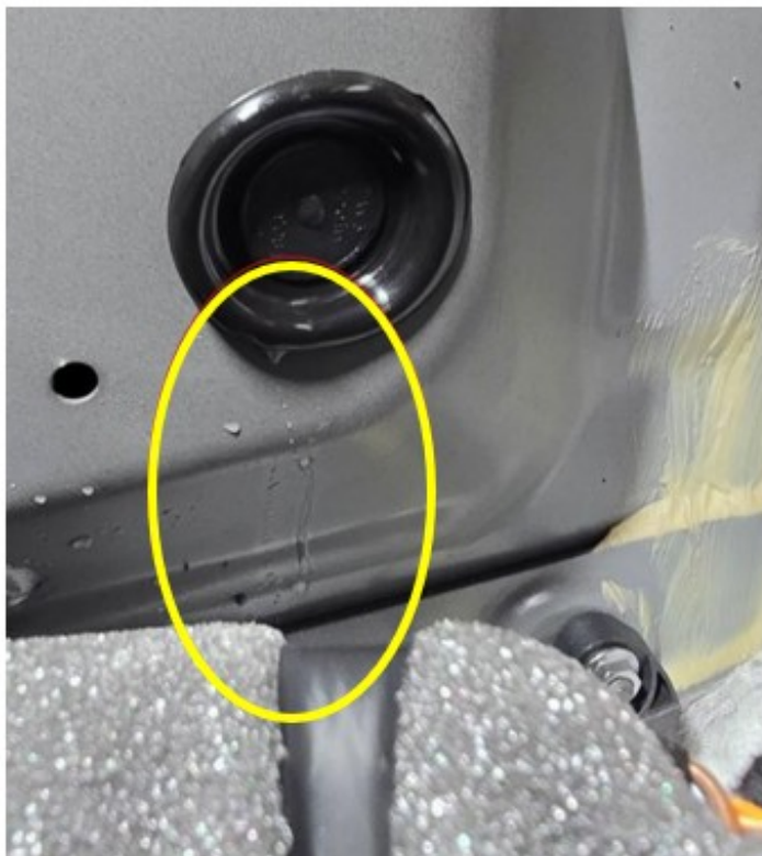
Figure 3. Sealing grommet with signs of leakage
