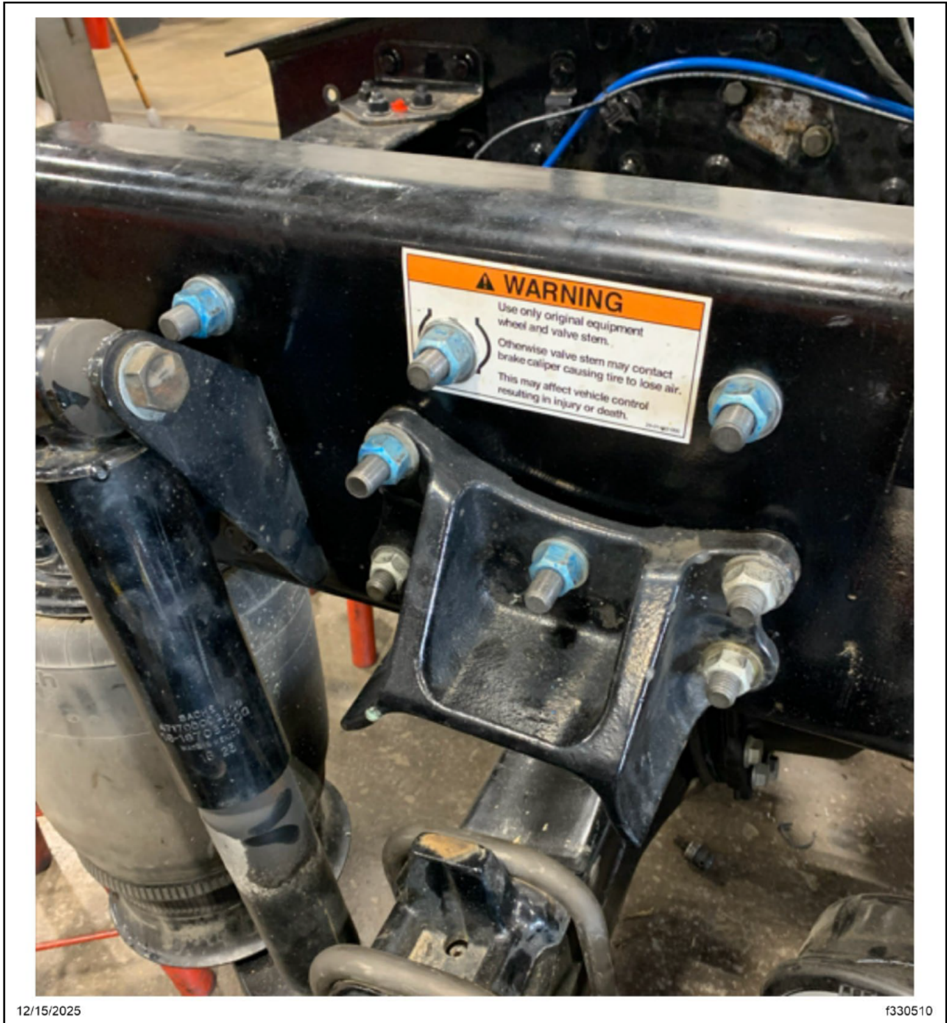
Fig. 8, Right-Hand Lateral Rod and Bolt Installation After Drilling Is Completed
