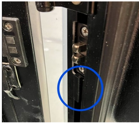
Step 15- Insert Screw At An Angle To Hold Sensor In Place. (You Can Also Super Glue)
