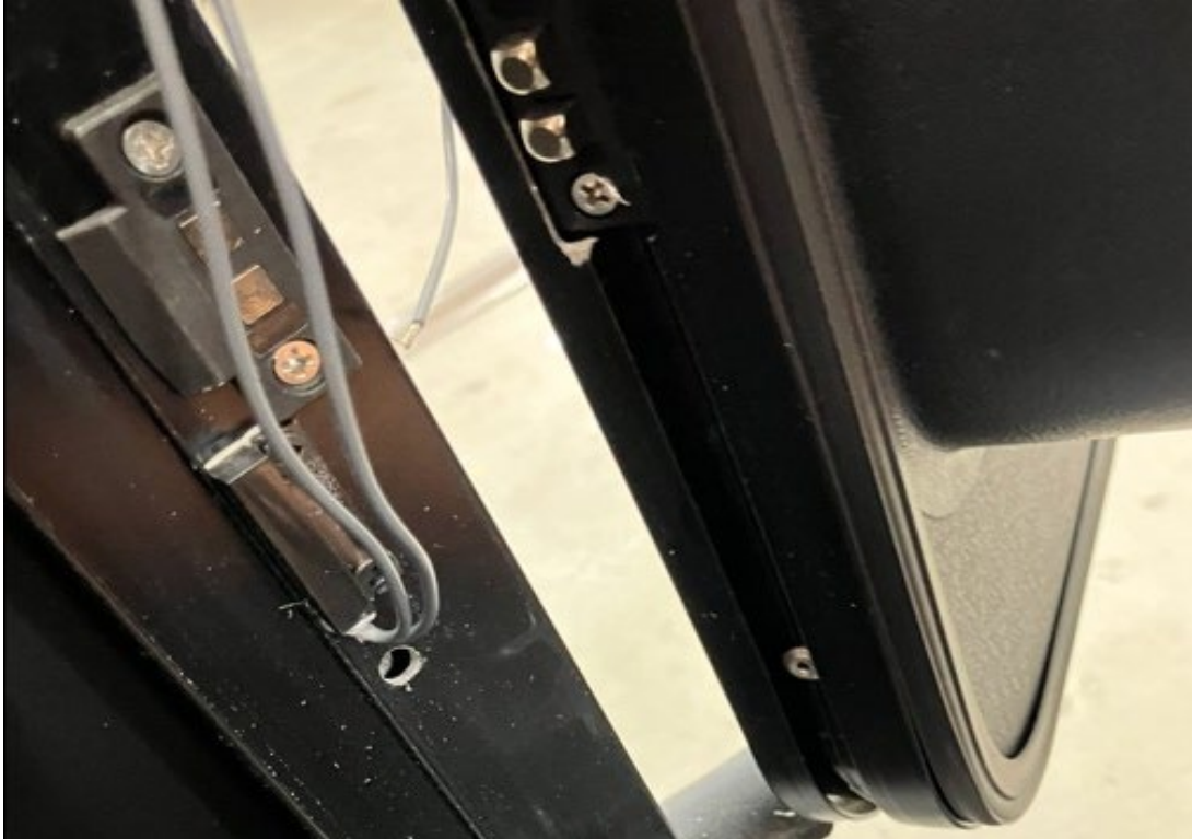
Step 11- Put Magnetic Sensor Wires Through Pilot Hole and Pull Wires Through.
