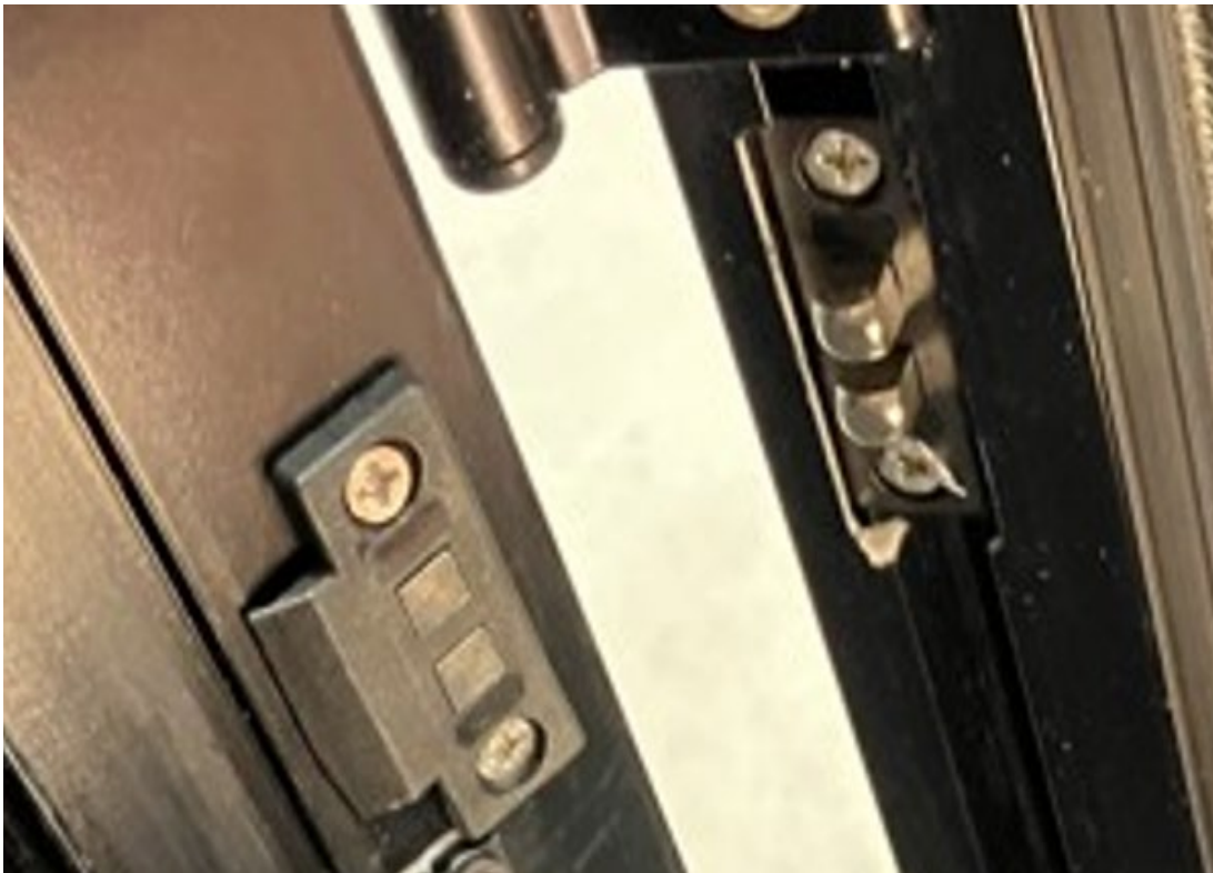
New Style Magnetic Sensor- Part # 591542
