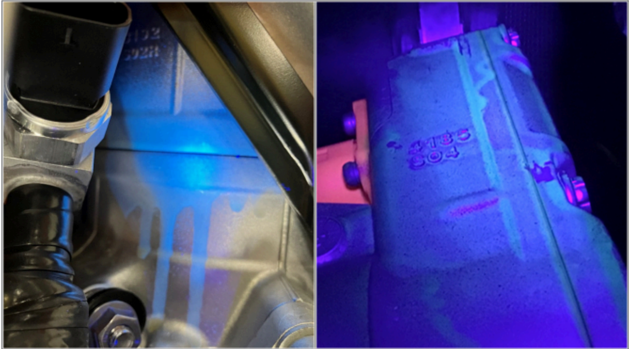
Traces of fluorescent corrosion preventive compound (example shown)
