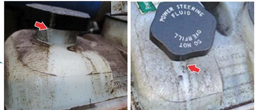
Acceptable misting of power steering vent
