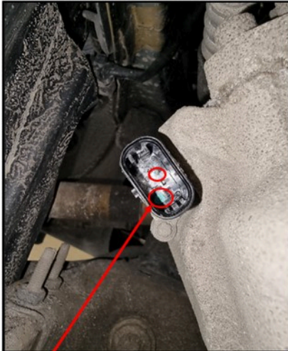
Oxidation in LV connector in ILK circuit pins (Check AC compressor and PTC heater)
