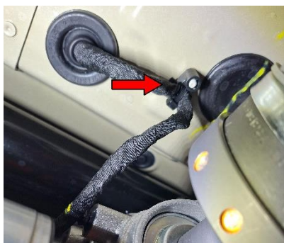
Figure 2 - Clip position and cable in correct position
