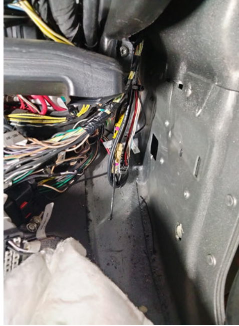
Fig. 9, Inspecting Drain Tube and Accessing Inner Cowl Structure
