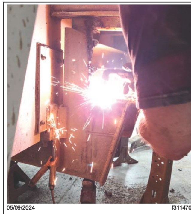
Fig. 29, Preparing for the New Rail Installation
