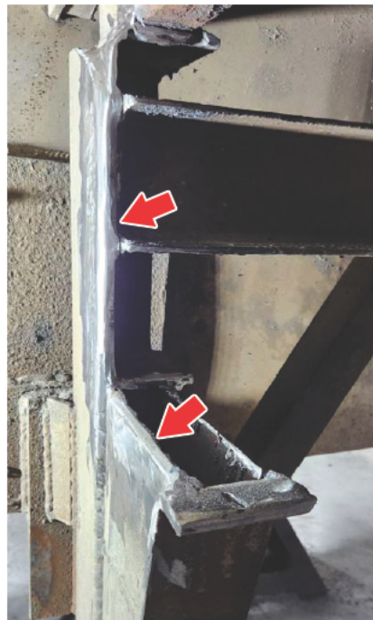
Fig. 31, Old Weld Cleaned and Prepared for the New Frame Rail Installation
