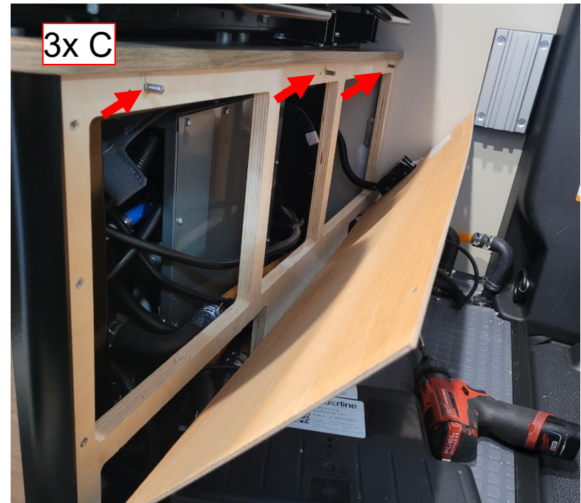
Figure 3: Riser removed and panel on the way out
