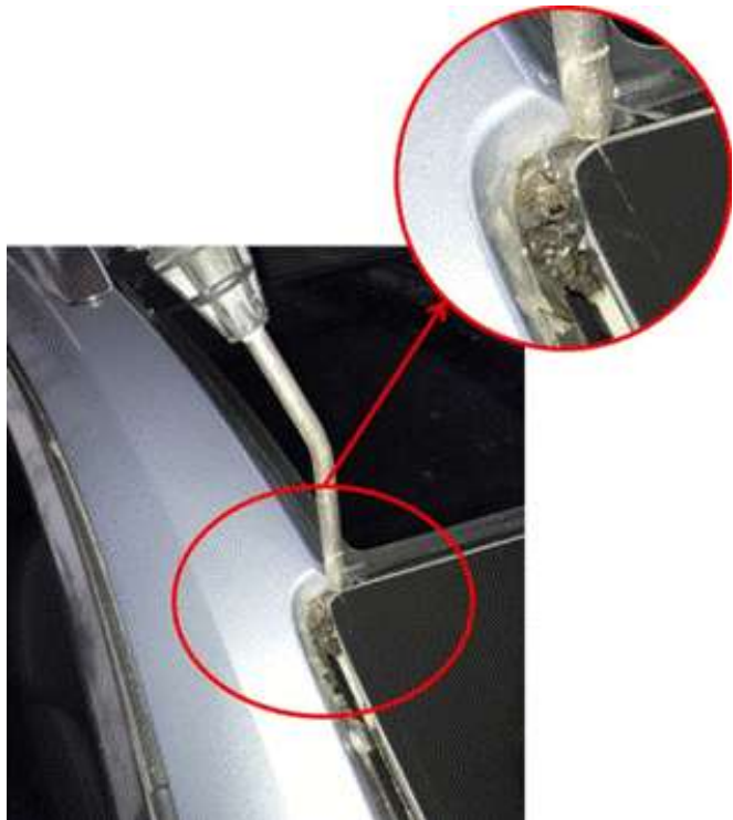
Figure 8. Removal of dirt and debris in the drainage channels using a pneumatic gun.
