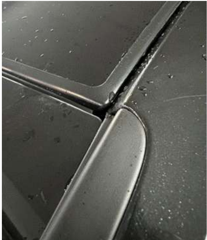
Figure 15. Water deflector reinstalled.
