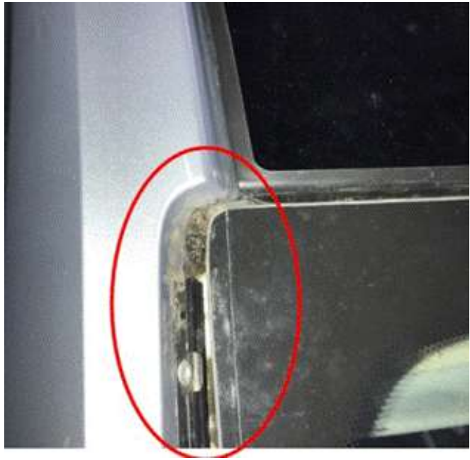
Figure 7. Dirt in exposed channel.
