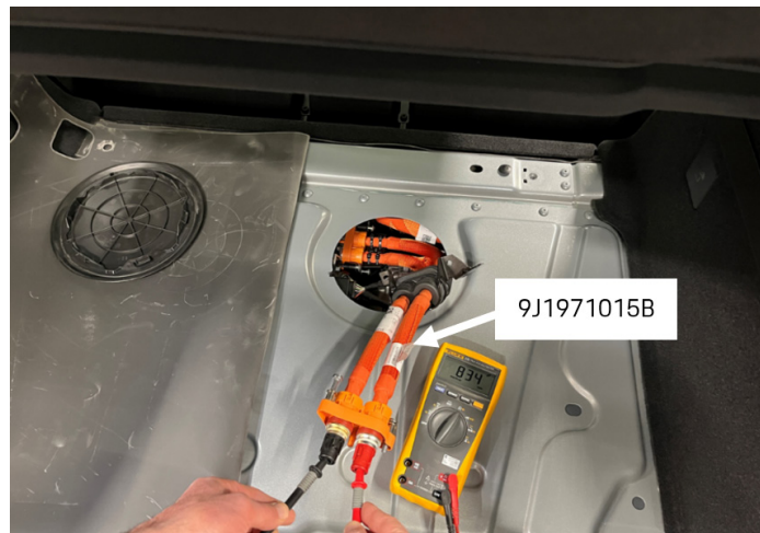
Figure 4 - Measuring Capacitance on Rear PE
