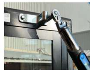
Torque to 9.7 - 10.7Nm
