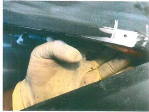
Apply Fibril to crack area and remove tape when it sets up
