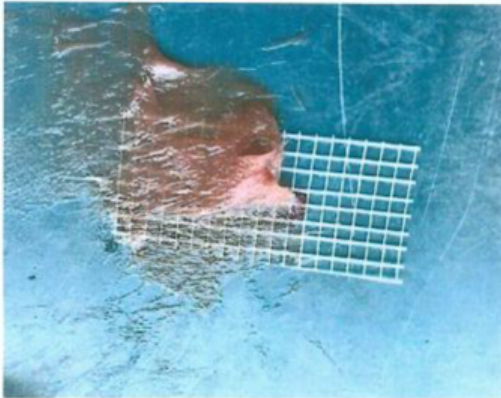
Apply Fibral mix to mesh tape
