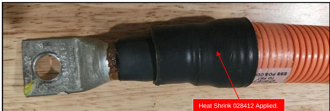
Figure 3 – Heat shrink applied over loom and lug heat shrink location reference.
