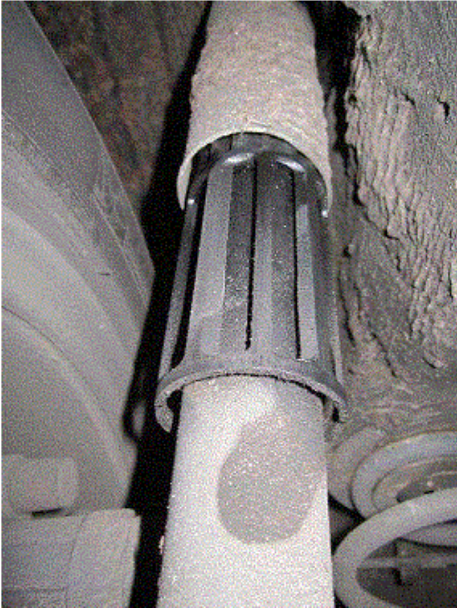
Figure 4) Not a leaking shock/strut
