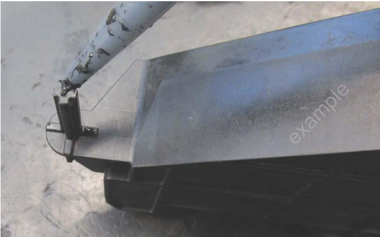
Figure 19. Lightly applying silicone sealant to the attachment point (example).
