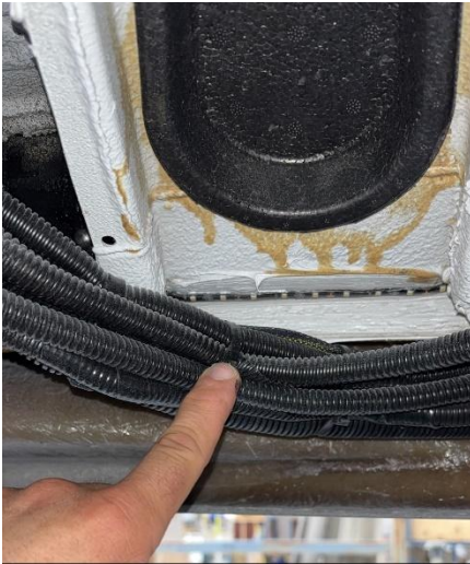
Step 1: locate wire harness with step lights
