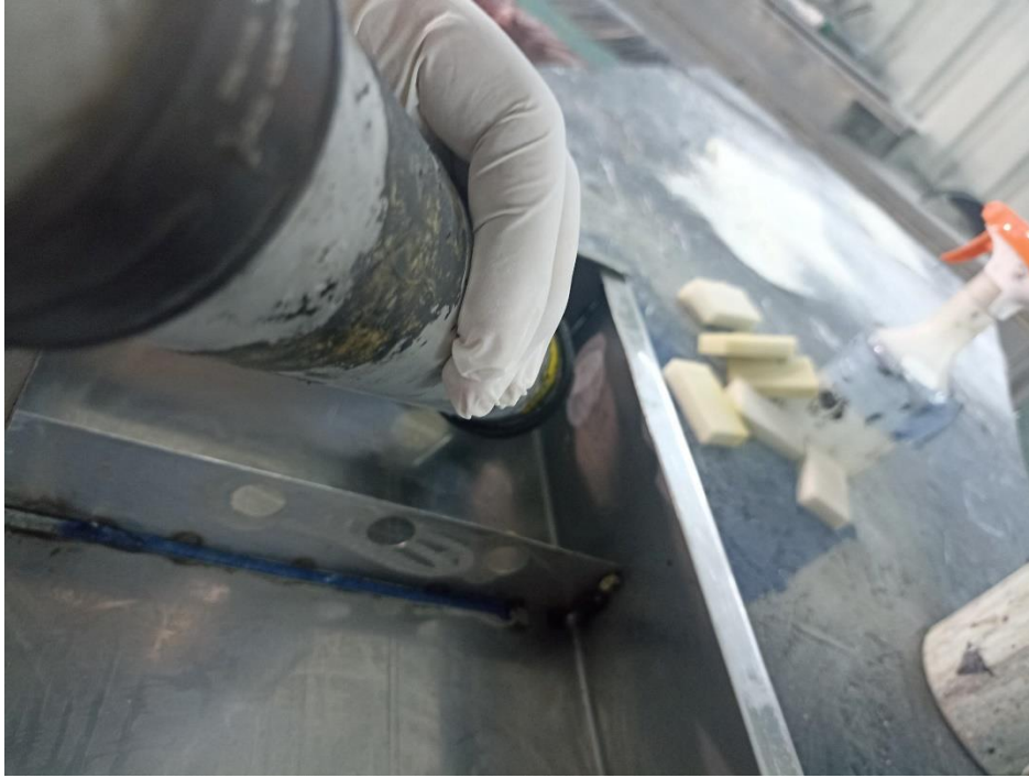
Figure 1 – Application of Sealing Compound
