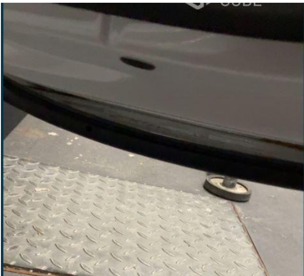
Figure 3. Door seal coming loose.
