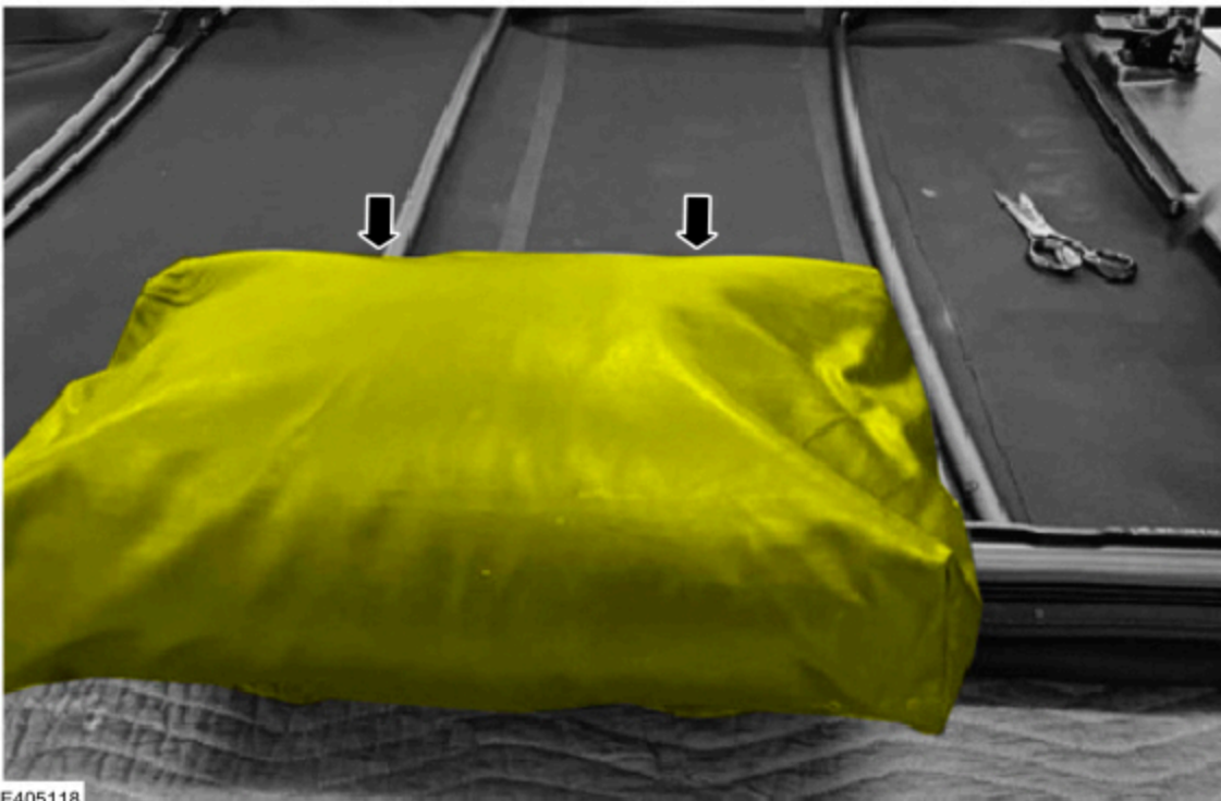
Figure 7 - Sandbag shown on top of frame hinge location. Left side shown, right side similar.
