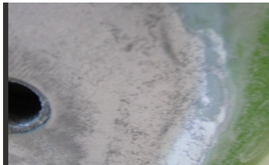
Pitting Found After Sanding Example (Fig. 1)
