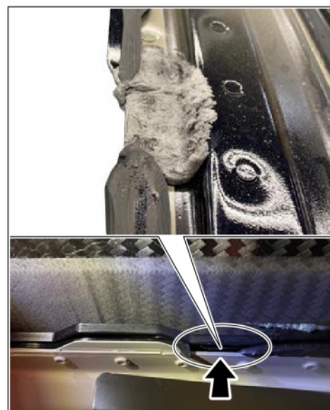
Bonding on roof module
