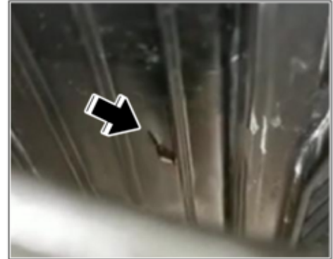
Crack in ATF pan
