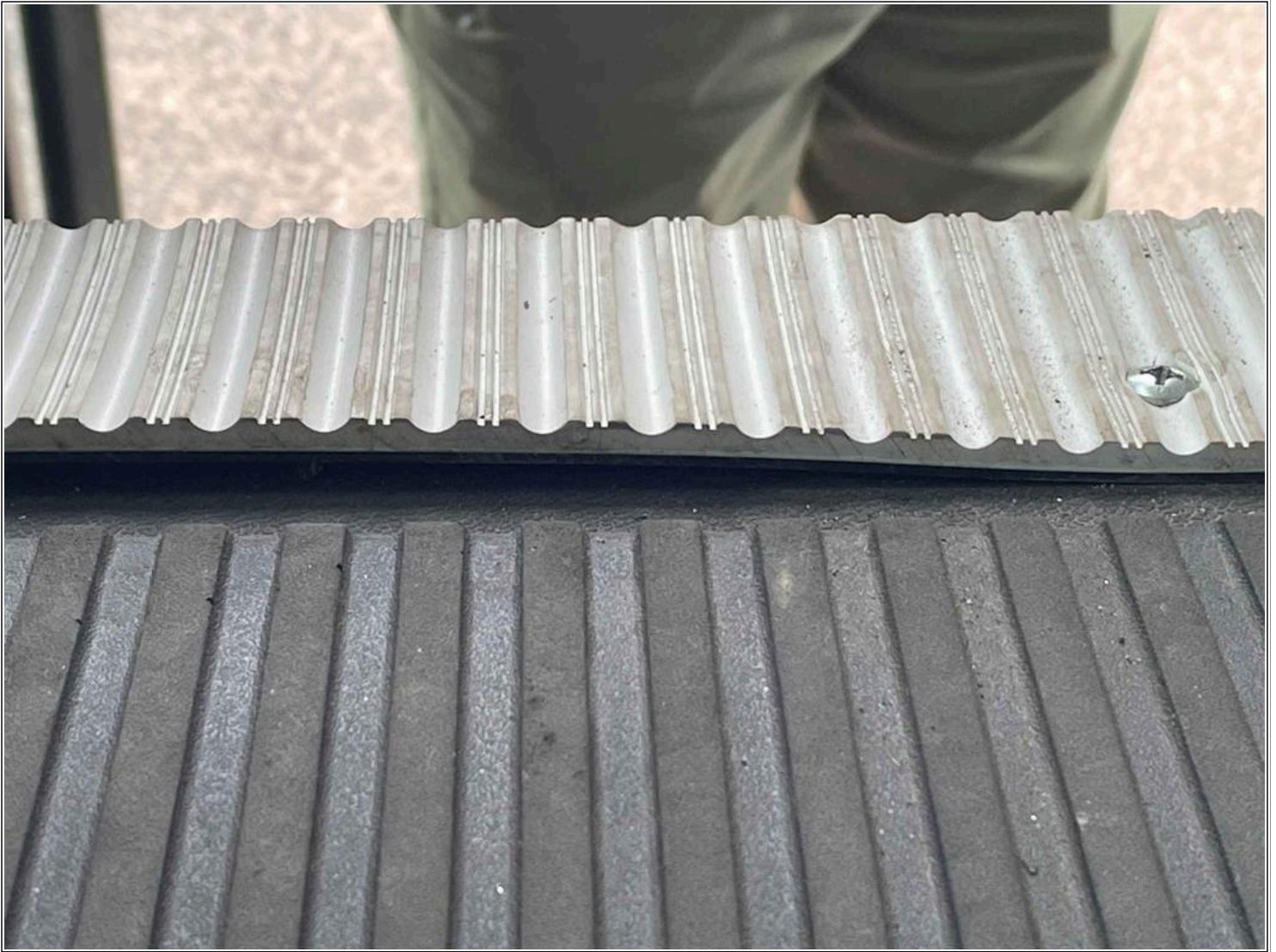
Figure #1: Step Tread Nosing Gap Example
