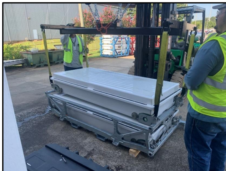
Figure 24: Rigging for Lifting Upper ESS Battery Pack Location Reference.
