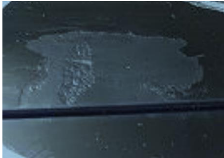
Damage caused by brake fluid
