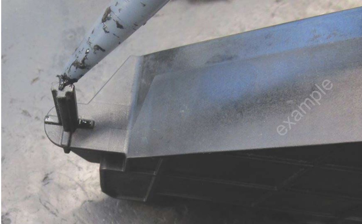
Figure 19. Lightly applying silicone sealant to attachment point (example).
