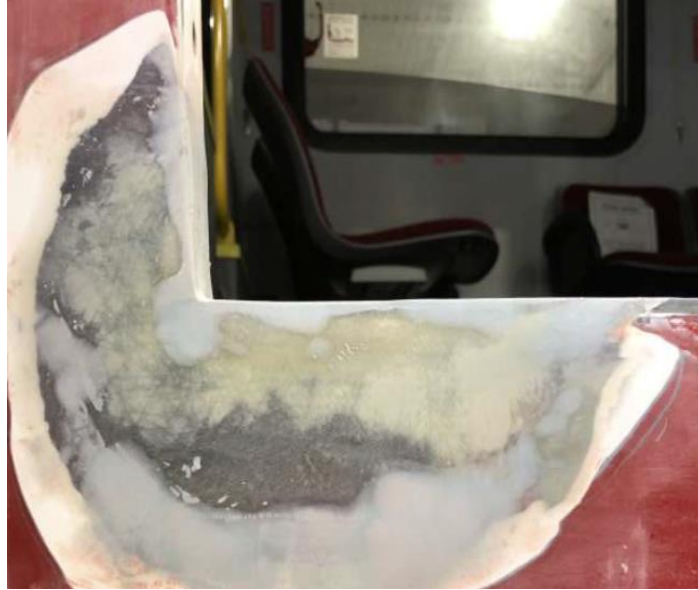
Figure 11 Filled and faired surface of the repair
