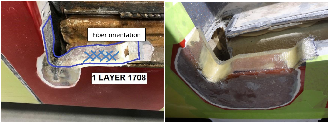
Figure 7 Application of first reinforcement ply (1708)
