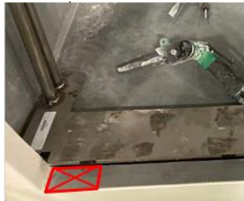
Figure 4 Drilling location for the crack repair
