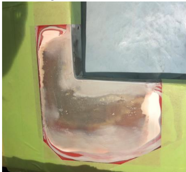
Figure 12 Masking the repair area prior to gel coating
