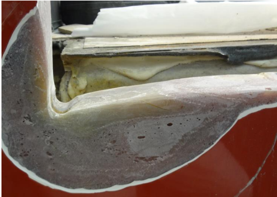
Figure 5 Excavated corner crack
