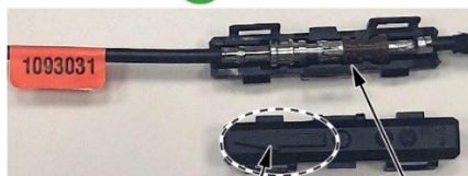
Arrow facing toward red flag label. Fully seated in splice box.
