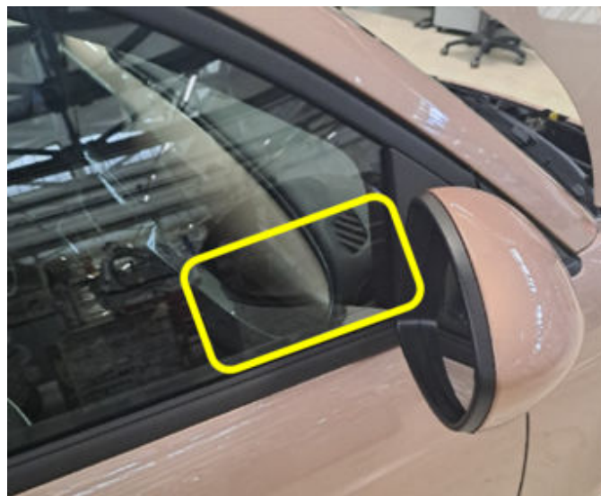
Fig. 1 Area To Water Test
