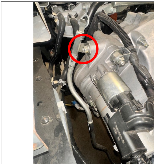
Figure 7 – Bolt Holding Oil Filler Tube
