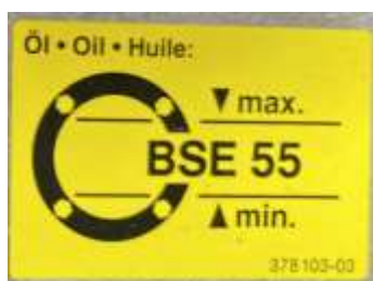
Figure 2: Oil level decal on the HVAC compressor
