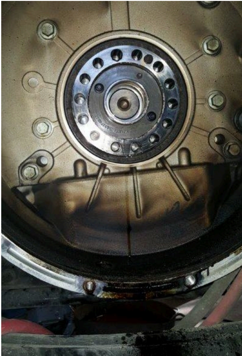
Engine Oil Leak - Not from Main Seal - Note that there is no oil path visible from the bottom of the crank flange down the face of the housing to the visible buildup
