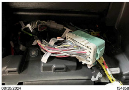
Fig. 16, Connector BHA Pulled Up into Area Behind the ICU for Access
