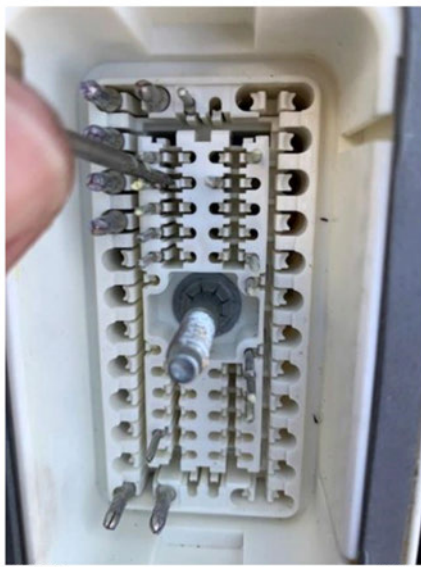
Fig. 9, Extracting the Terminal
