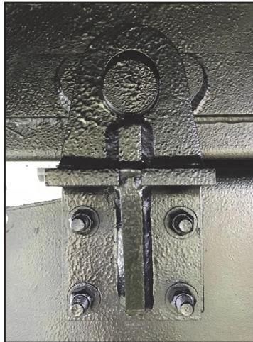
Figure 6. Rear Mounting Pin Weldment Installed and Painted
