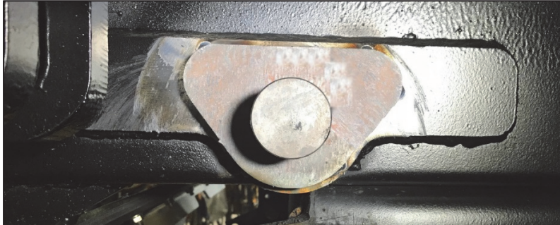
Figure 5. Pin Mounting Weldment Tack Welded onto Original Mount Plate
