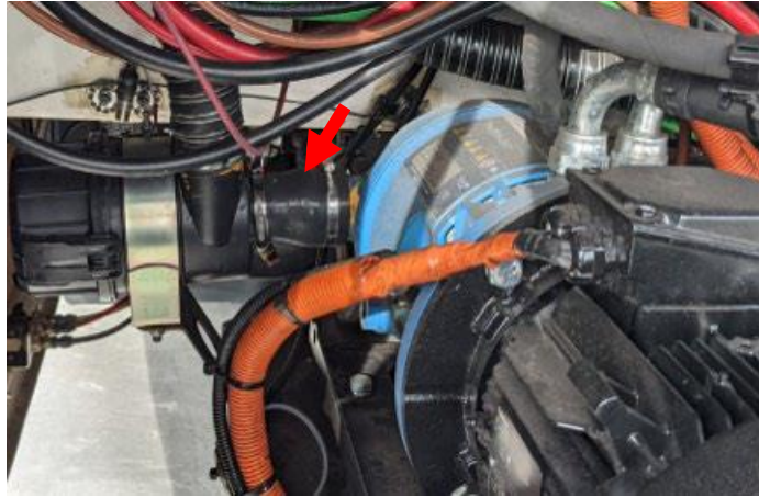
Figure 14: Air Compressor Old Coupler
