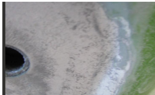
Pitting Found After Sanding Example (Fig. 1)
