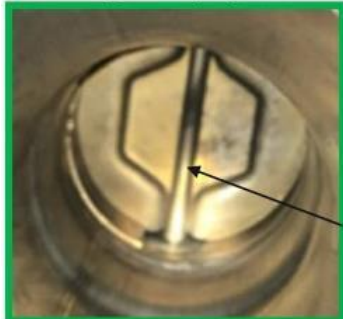
OK mounting of valve group show this visible shaft:
